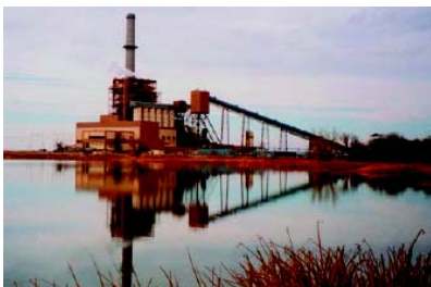
Figure 4. Xcel Energy's Pawnee Power plant at Fort Morgan, CO.
