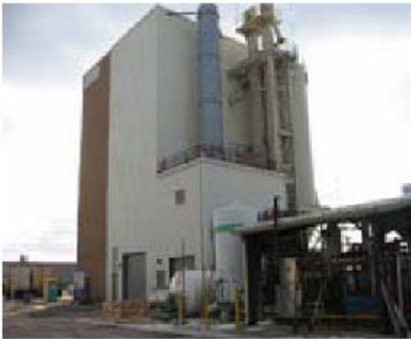
TDA sorbent is qualified for Siemens' UltraClean™ Process at GTI's 10 ton/day FlexFuel Gasification Facility (Plains, IL)
